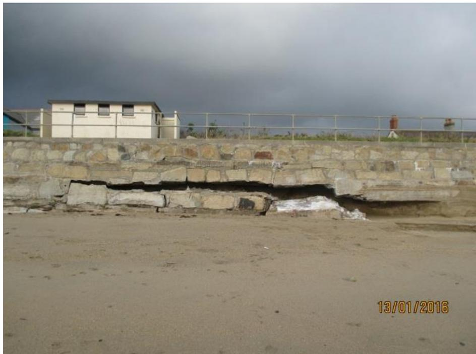
**Figure 1** Damage to the seawall at Long Rock in the aftermath of Storm Frank, January 2016
