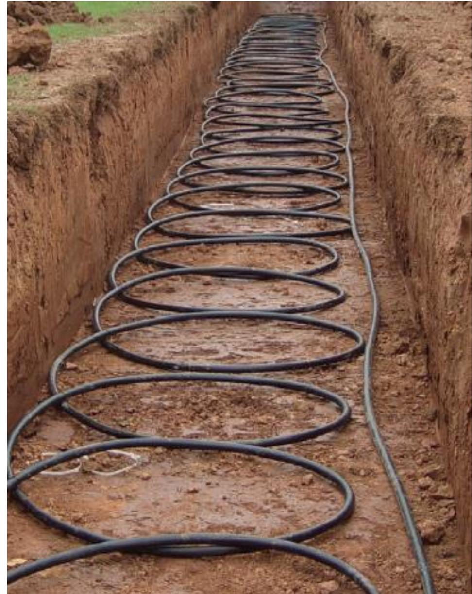
Pipework laid in a trench for heat pump installation. Photo courtesy of Community Energy Plus.
