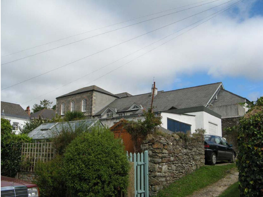
South elevation of the former Market Hall and the 1991 extension
