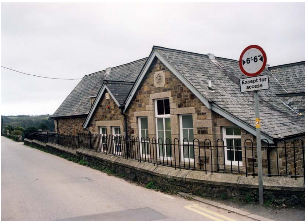
Devoran School from the north (St John's Terrace)
