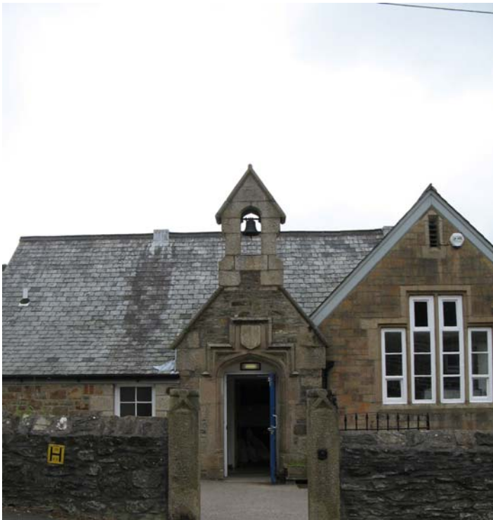
Detail of JL Pearson entrance facing Market Street
