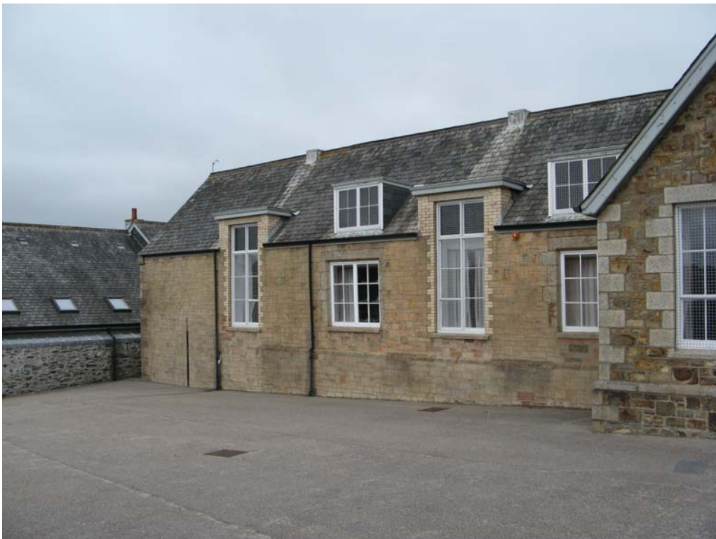
East elevation facing the playground
